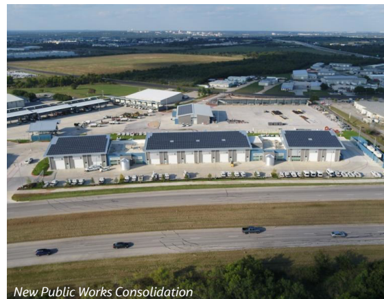
New Public Works Consolidation
