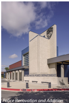
Police Renovation and Addition
