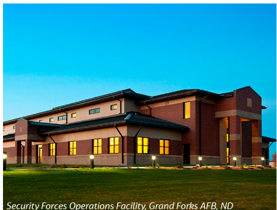
Security Forces Operations Facility, Grand Forks AFB, ND
